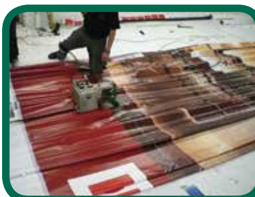
Track Welding on Floor
